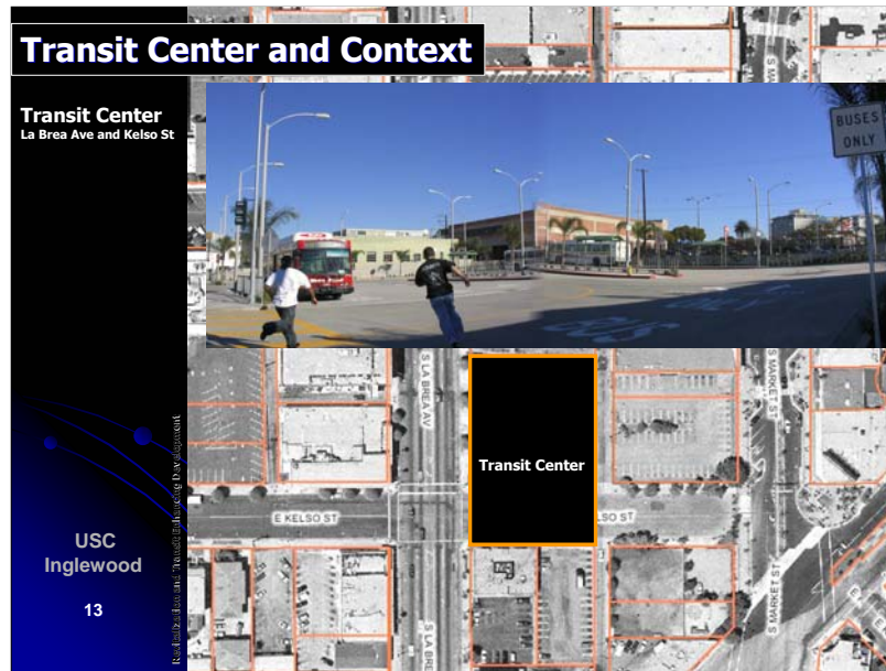
View of the transit center at the intersection of La Brea Avenue and Kelso Street.
