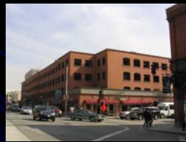
Parking Structure, Alhambra, California
