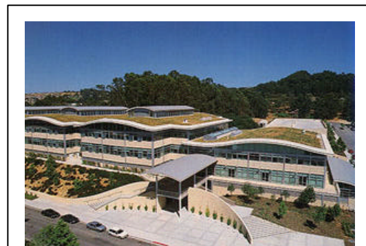
Picture 6: Gap Headquarters (topography) Source: www.ecotecture.com
